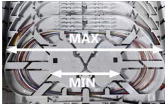
6.2.2. Route the fiber throughout the groove plate to the dedicated splice trays.
