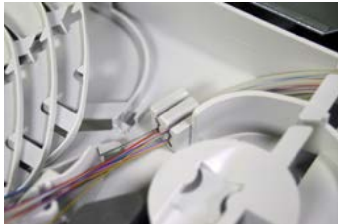
6.1.9. Push and click the tube holder into the tray. Rout the transportation tubes into the FACT element.
