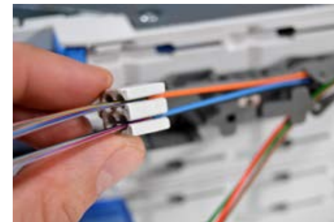
7.1.3. Slide on the tube holder.
