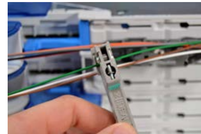
7.1.2. Strip the loose tubes at the marked point and clean the fibers.
