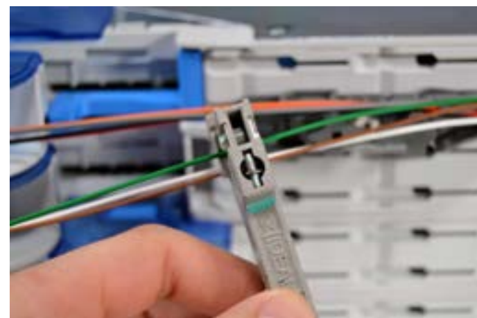
6.1.2. Strip the loose tubes at the marked point and clean the fibers.
