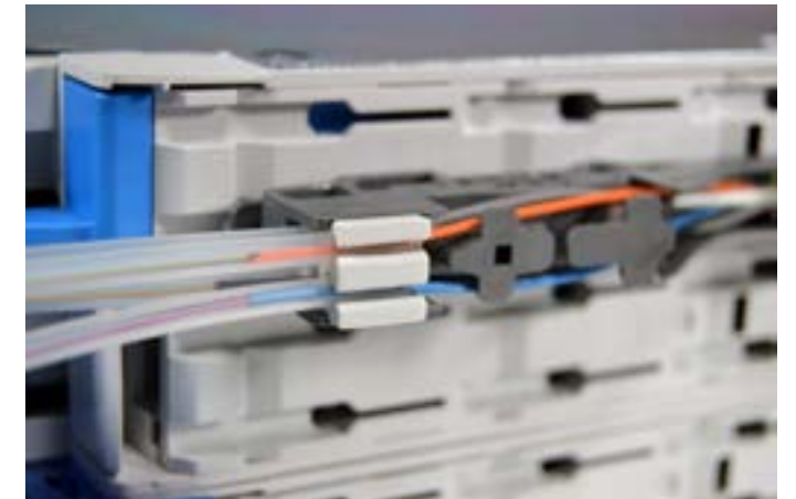
6.1.6. Slide the transportation tube in the tube holder. Make sure that the transportation tube is pushed in, until the end.
