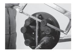
14.2 Remove any dirt, mud or other contaminants from the cable sheath for approximately 2 meters with a clean cloth. Take the cable seal sleeve from the kit FOSC-B/D-CSEAL-1-NT and slide it over the cable. The non-coated edge of the sleeve and the arrows should be pointed to the base of the closure.
