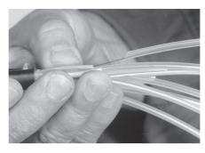
5.4 Align cable ring cuts with edge of base. Slide strength members into clamps and tighten. Cut away the excess length of strength member.
