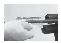
14.10 Slide the cable seal over the port and shrink the cable sleeve on the base side with the recommended hot air gun device. Use the reflector to ensure heat
