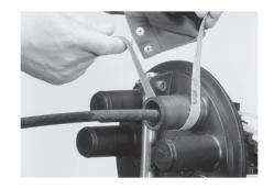
14.8 Place cable seal over the drop outlet of FOSC base. When cable seal butts against the base, mark the sleeve length on cable sheath.
