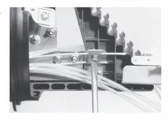
5.5 If required, connect shield continuity wire of both cables with shield continuity clip. Talk pairs, if present, will be connected together according to the local procedures.
