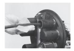
14.7 Abrade port and cable sheath circumferentially on the cleaned area with the abrasive strip. Remove any abraded material with a clean cloth.
