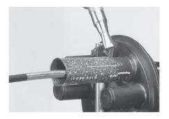
14.11 Shrink down the end of the sleeve on the cable side. Heat till the sleeve shrinks down onto the cable and the green thermo-indicating paint is converted to black. A ring of red adhesive should be visible at the cable on the end of the sleeve.
