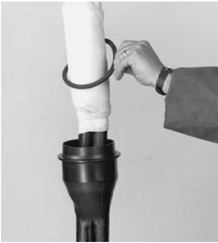
15. Before installing the sealing ring on the base part, ensure the sealing ring area is free from dirt.
