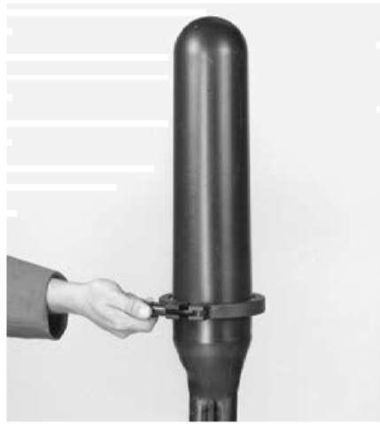
16. Put the dome in place over the joint and tight the two parts together with the clamp.
