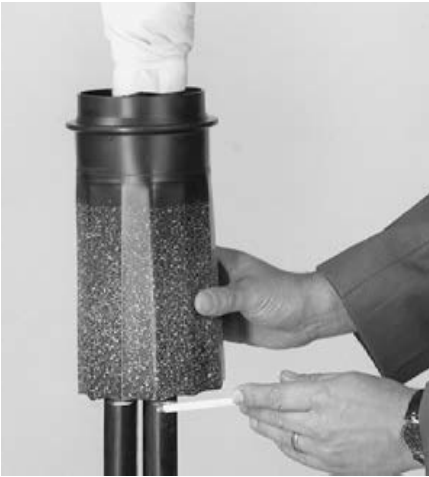
4. Slide the base part over the joint such that the cable jackets are protruding a thumb width ( \pm 2.5 cm). Above the base part and mark the end of the base part on the cables. Remove base part.
