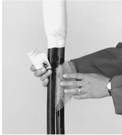
2. Remove solvent impregnated tissue from its package and clean the cable over a distance of \pm 25 cm.
