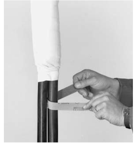
3. Abrade the cables over the cleaned lengths.
