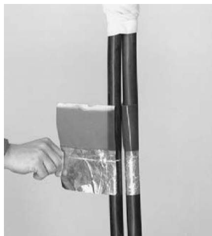
7. Apply cable wraps around each cable. Line up the aluminium of the cable wrap with the marks on the cables.
