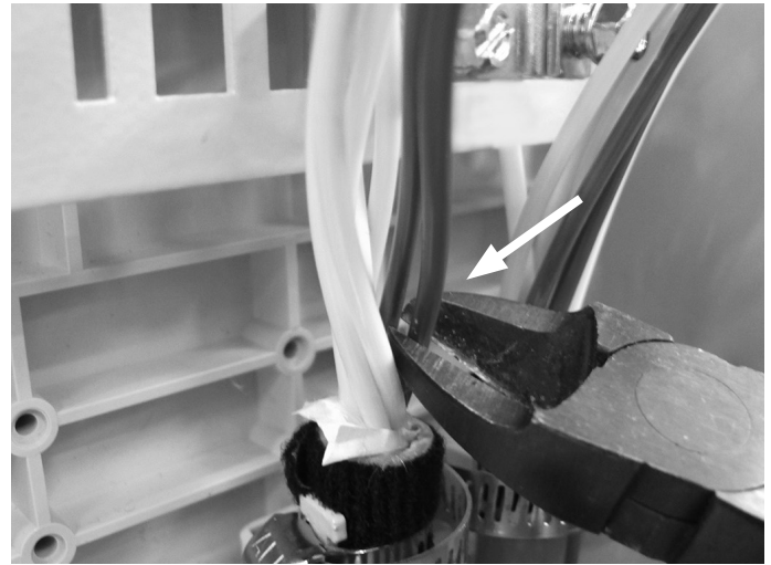
8.16. Cut the required loose tube at the jacket end for a looped cable or take out the required loose tube for a stubbed cable.
