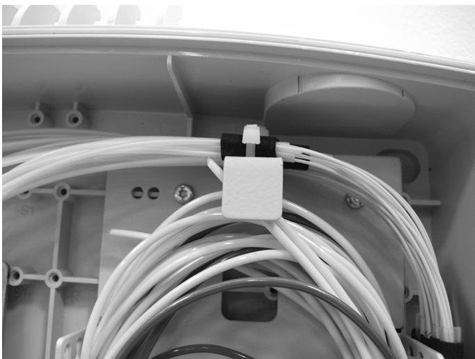
13.8. Two bundles of up to 12 tubes can be secured to the loop basket. When attaching the first bundle, make sure the second one can still be easily secured to the loop basket.
