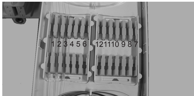
14.1. Splice the drop fiber to the feeder splice per standard practice and store the splice sleeve in the splice module. Following the sequence of the splice sleeves in the splice module as shown above.
