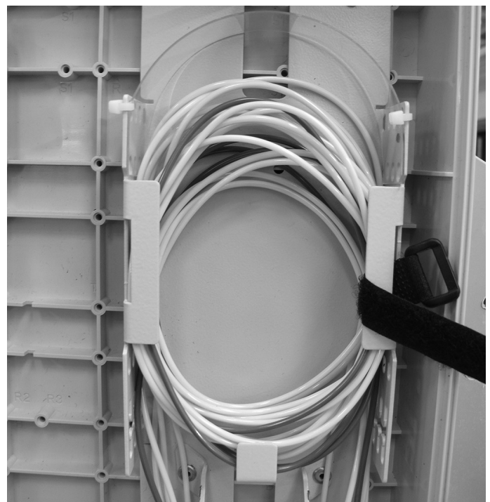
8.17. Remove the Velcro, hinge the trays down, and store the feeder tubes in the storage basket.
