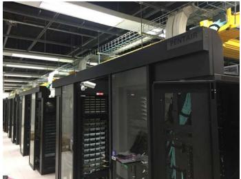
• The vertical cable management system, installed in standard cabinets, did not require any horizontal space—increasing the density of power distribution cabinets and main distribution cabinets by approximately 80 percent
