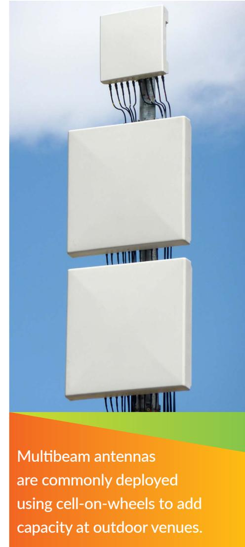
Multibeam antennas are commonly deployed using cell-on-wheels to add capacity at outdoor venues.
