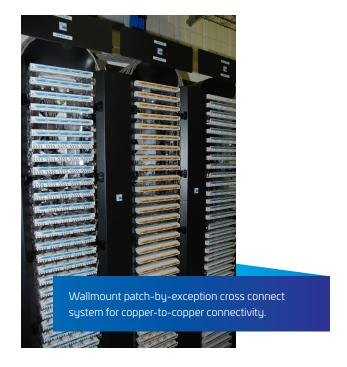
He said the network had sufficient bandwidth to fulfill the airport's requirements for the next 5-6 years. In addition, the Category  $6_A$  HighBand 20 patch-by-exception cabling system allows the Melbourne Airport IT team to easily install additional cable modules without undertaking any work on the cable support systems.
